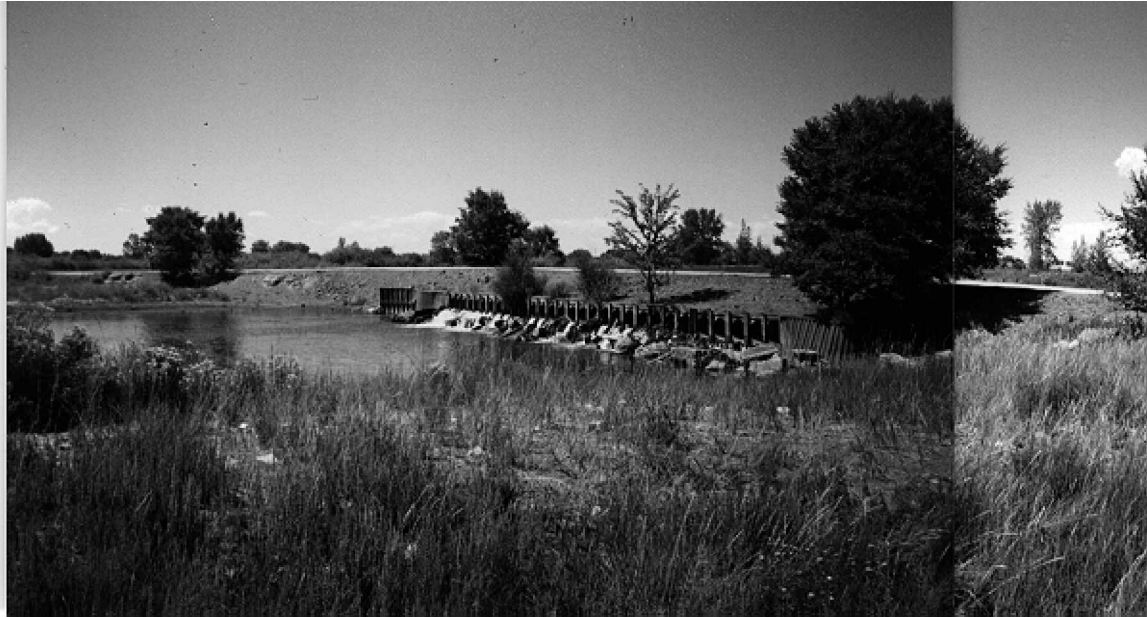
Chicago Ditch Diversion Dam on the Rio Grande River
